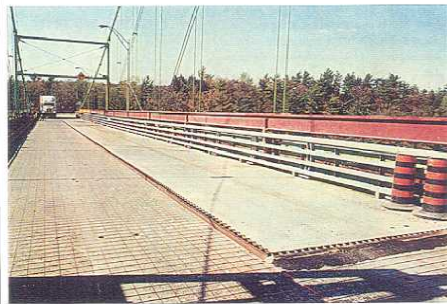
NIGHT CREWS WERE ABLE TO REPLACE 102 SUSPENSION SPAN DECK PANELS IN JUST 62 DAYS, BEATING CONSTRUCTION SCHEDULE REQUIREMENTS WHILE KEEPING BOTH LANES OPEN DURING THE DAY.
