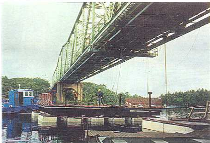
WORK PLATFORM SECTIONS WEIGHING 60 METRIC TONS EACH WERE FLOATED ON POLYSTYRENE, PULLED BY TUGBOAT BENEATH THE OVER-WATER SPANS (ABOVE) AND THEN LIFTED INTO PLACE (BELOW).
