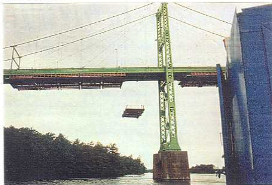
WORK PLATFORM SECTIONS WEIGHING 60 METRIC TONS EACH WERE FLOATED ON POLYSTYRENE, PULLED BY TUGBOAT BENEATH THE OVER-WATER SPANS (ABOVE) AND THEN LIFTED INTO PLACE (BELOW).
