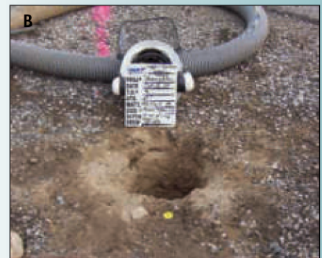
A: Vacuum excavation equipment at the Hwy 401/Homer Watson Blvd. project. B: A test hole installed on a utility structure. Photos courtesy of Lawrence Arcand, TSH/TBE Subsurface Utility Engineers.
