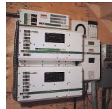
A bank of batteries stores energy, while two inverters are required to convert wild current to household electricity.
