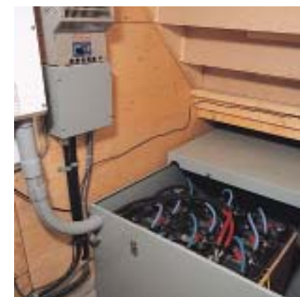
A bank of batteries stores energy, while two inverters are required to convert wild current to household electricity.
