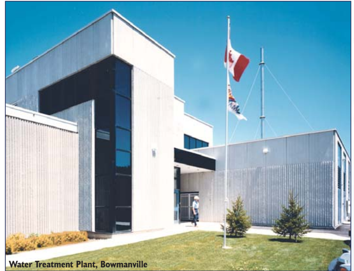
Water Treatment Plant, Bowmanville
