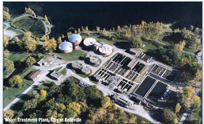
Water Treatment Plant, City of Belleville
