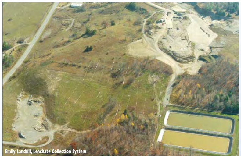
Emily Landfill, Leachate Collection System
