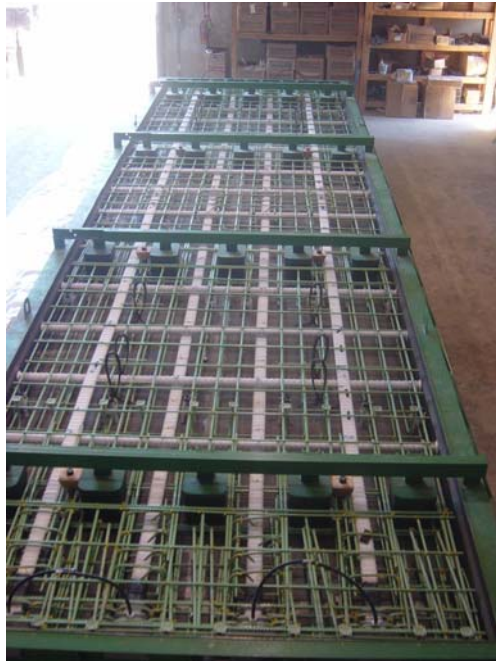
Figure 7: deck panel ready to be cast
