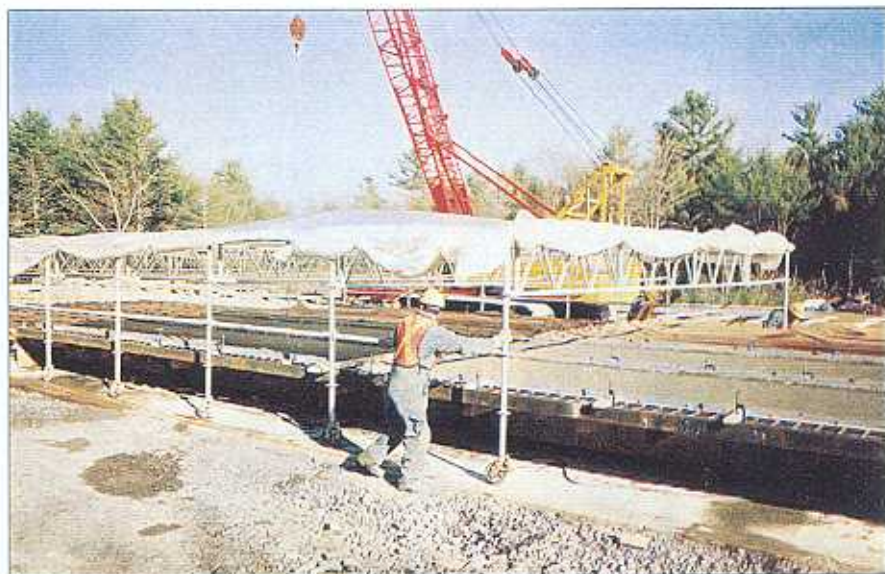
Positioning the polyethylene canopy over the freshly-poured concrete.
