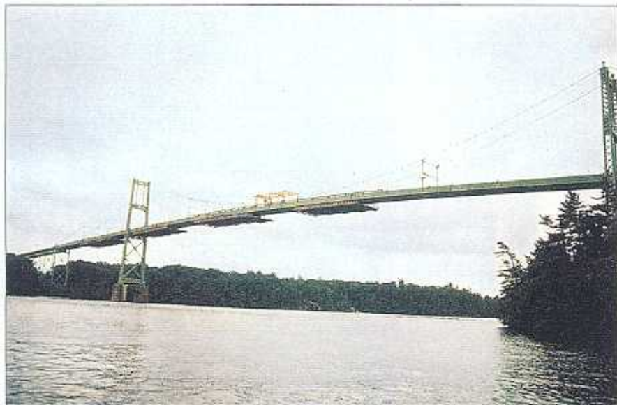
Suspension spans with work platforms and portal frame gantry.
