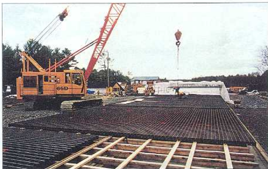
Placing the steel-grid deck panels on the casting table.
